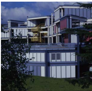
Ecole d'archit. Nanterre © Joly / Cardot
