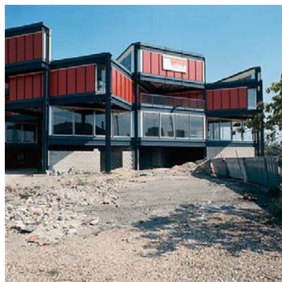
Ecole d'archit. Nanterre © Joly / Cardot
