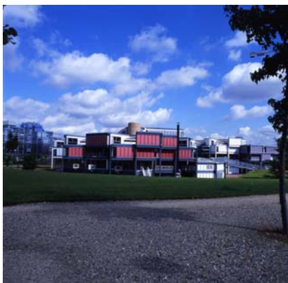
Ecole d'archit. Nanterre © Joly / Cardot
